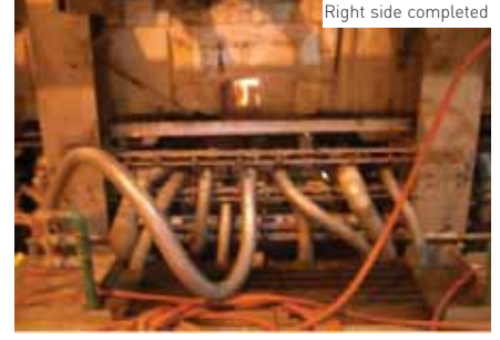
Right side completed
